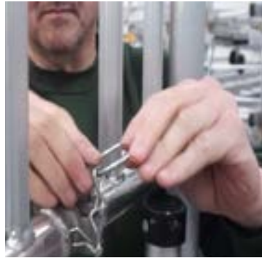
Place the pin through rear gate to secure
