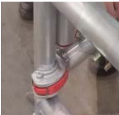
Attach bottom rear brace claw to the other side
