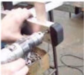
1.Drill Rivets
