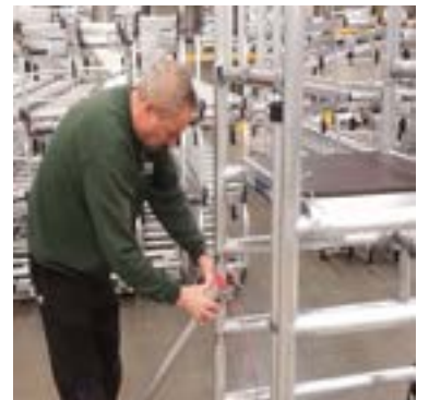
Attach and tighten both stabilisers
