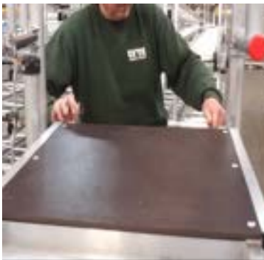
Clip the deck onto the side frames.
